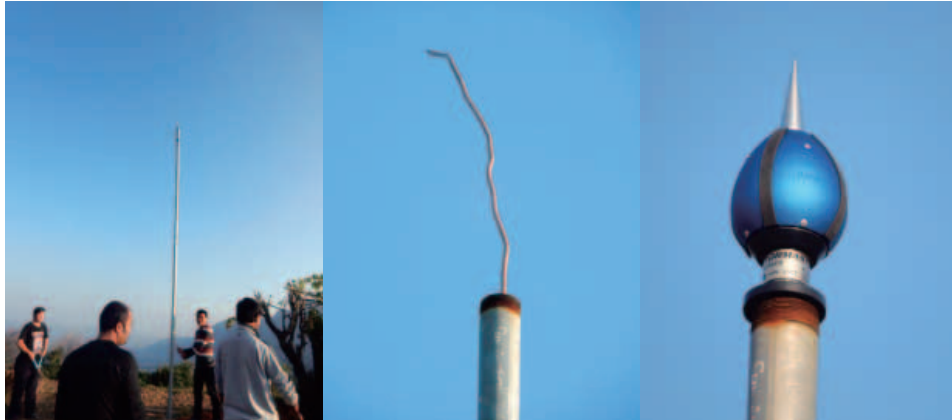
Figure 38 : Installation of Lightning Arrestor
