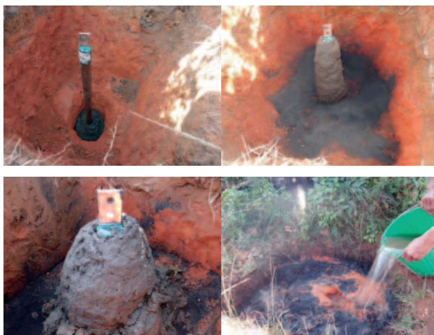
Figure 37 : Lightning Arrester
